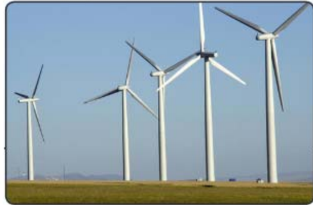
Figure 3: Large wind farm example
