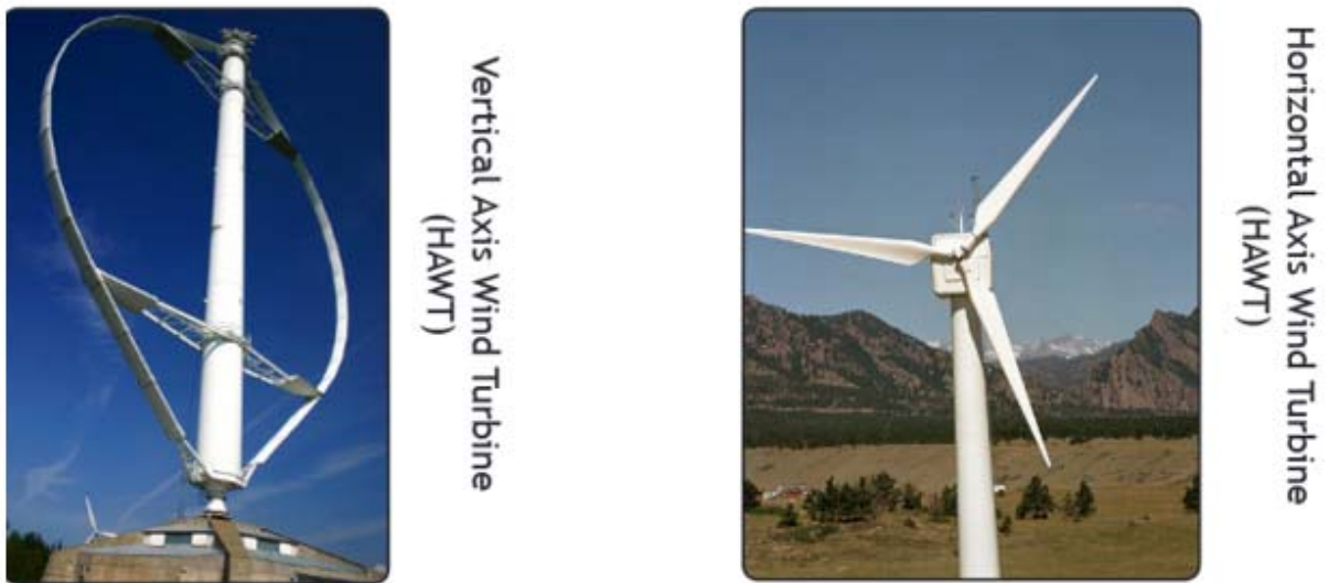
Figure 2a: Two main wind turbine categories
