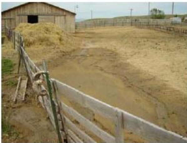
Photo 3. Signs of OLF initiated from roof runoff 6/12/06
